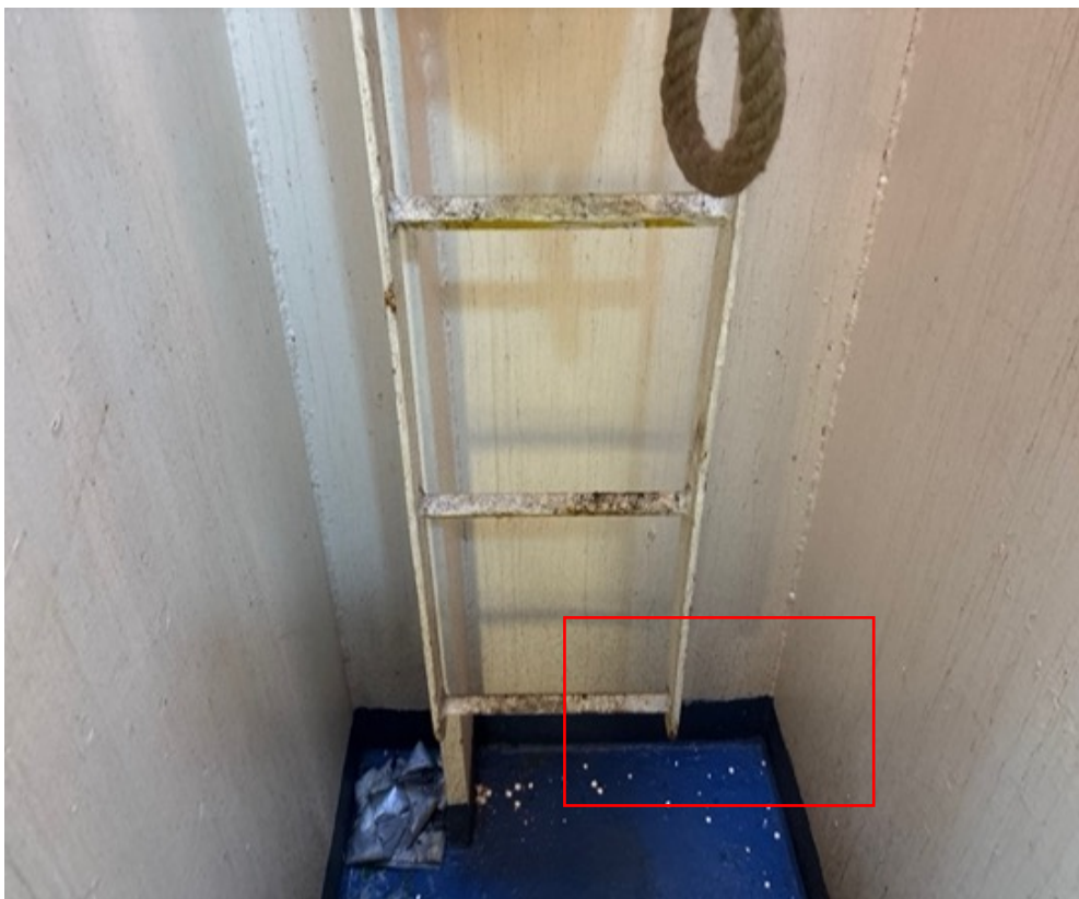
Broken emergency exit ladder
