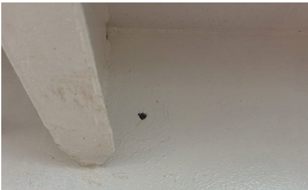
Hole in the forecastle space aft bulkhead
