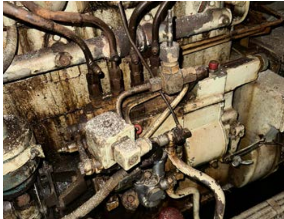
Oil leakage in emergency generator
