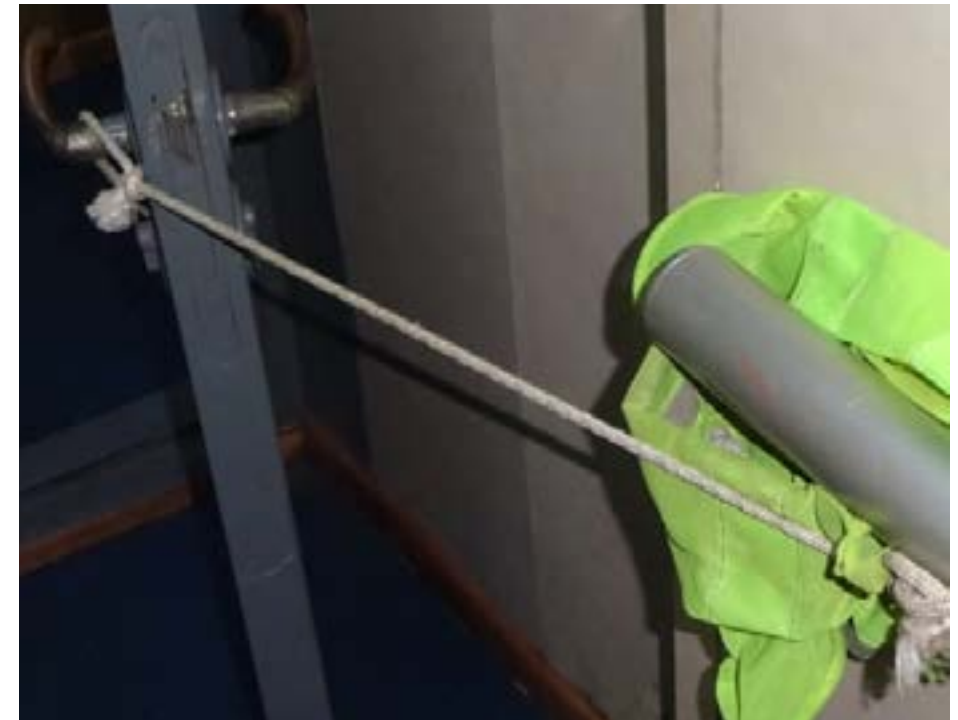
Fire door fixed with rope
