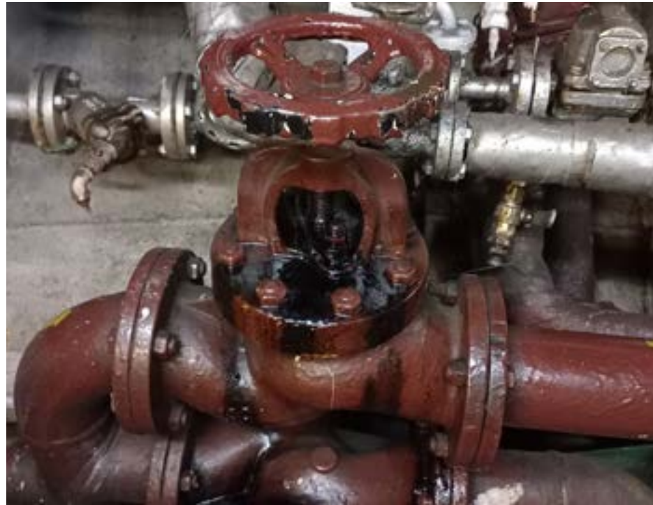
Fuel leakage from valve handle
