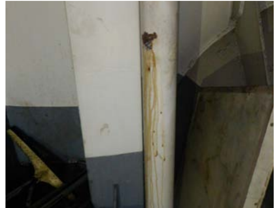
Holes on air vent' pipes due to heavily corrosion
