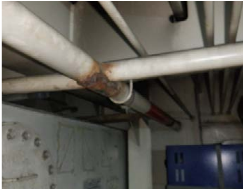
Temporary repaired pipeline with doubler plate
