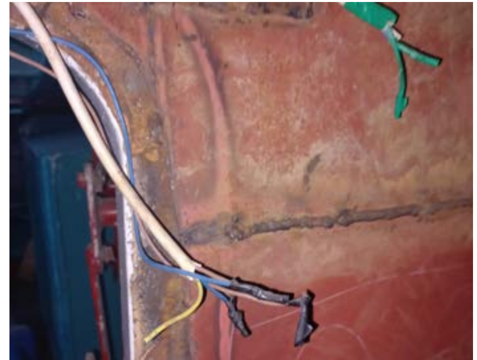
Open electrical cables in engine room
