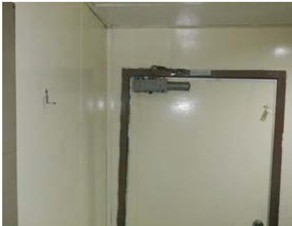
Fixed fire doors with hooks, cables etc.
