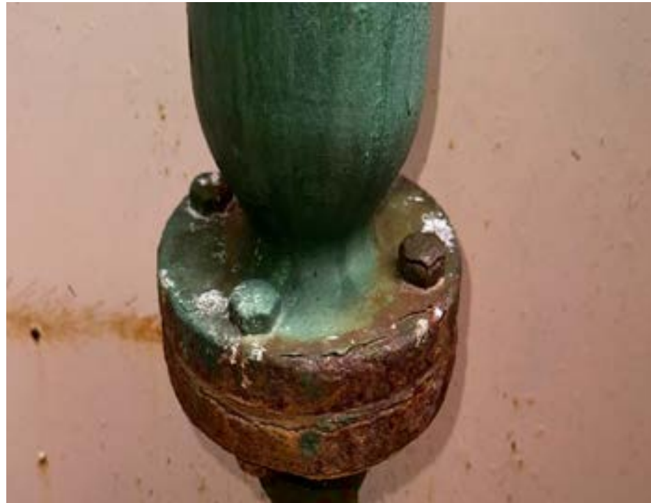
Corroded air ventilation
