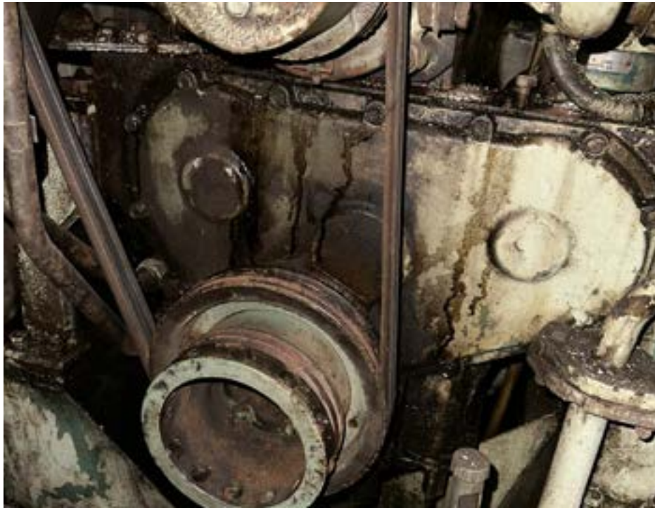
Missing cover of pulley of emergency generato
