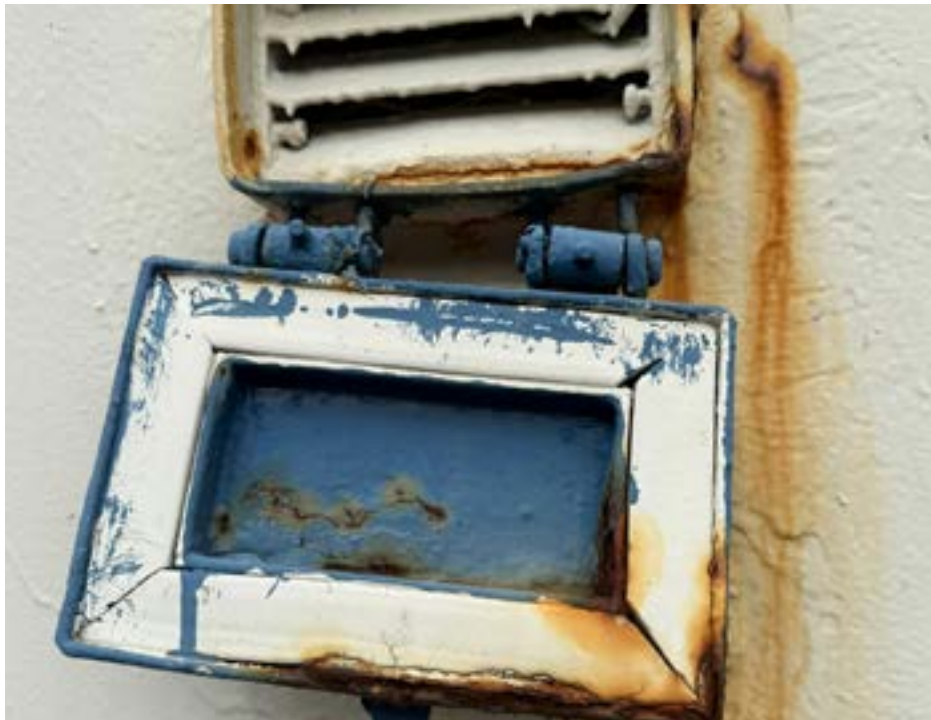
Defected ventilation hatch cover
